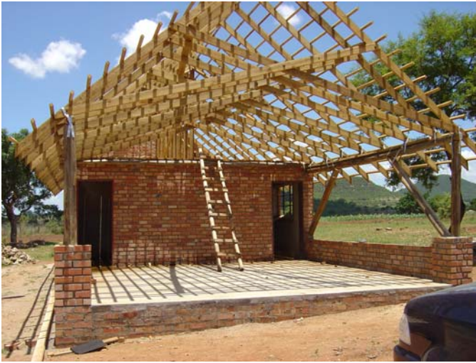
A KaGogo Social Centre being built by the community.
